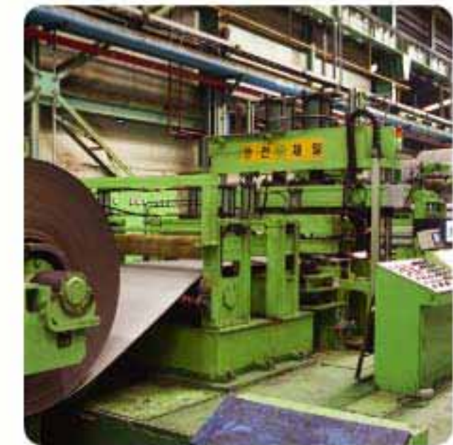
• Build up Line
